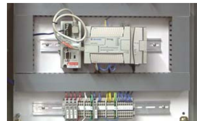
Typical Indicator Unit with Touch Screen Operator Interface. Allen-Bradley PLC ML1200 with DH485 Interface Module.
